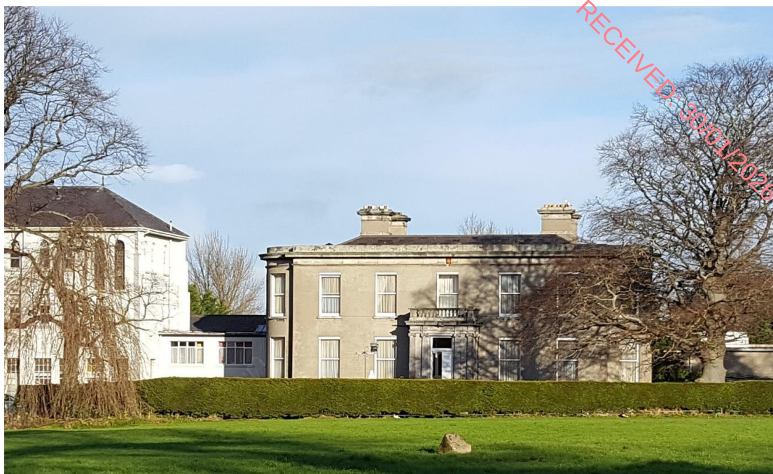
Figure 17.8 - View from South-west (pre-2021 demolitions)
