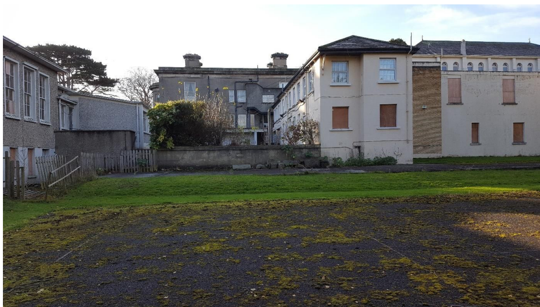
Figure 17.7 - View from North-east (pre-2021 demolitions)
