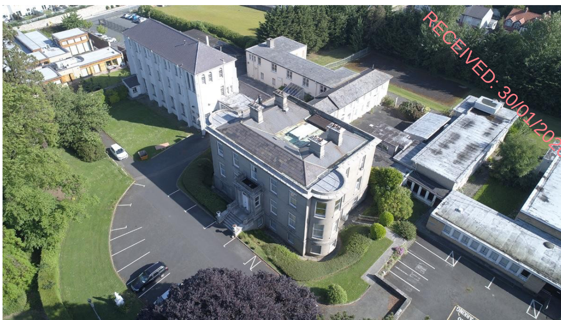
Figure 17.6 - Aerial view from South (pre-2021 demolitions)
