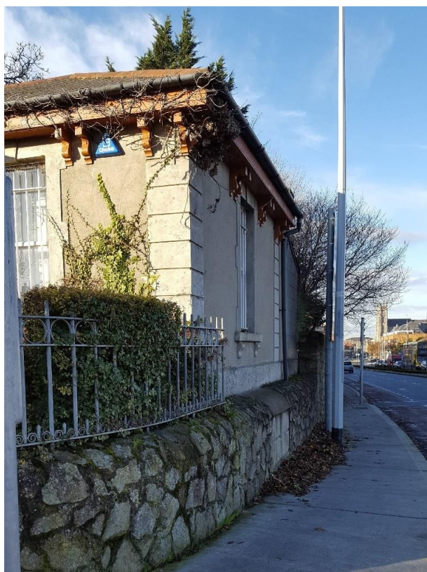
Figure 17.10 - New boundary wall
